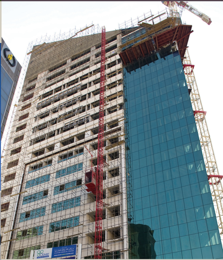
▲ A shot of the Building during construction
